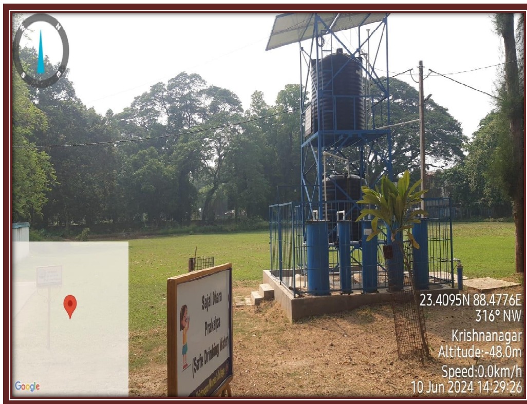
Fig. 15 : 'Sajal dhara' after installation
