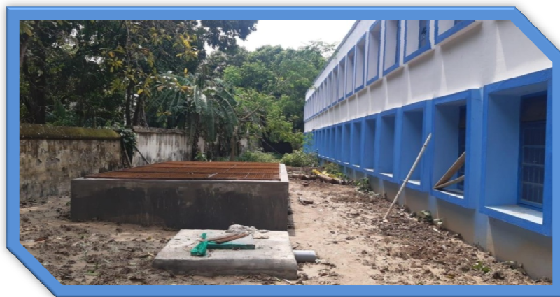
Fig. 12 : Rain Water Harvesting Project's Site in Campus
